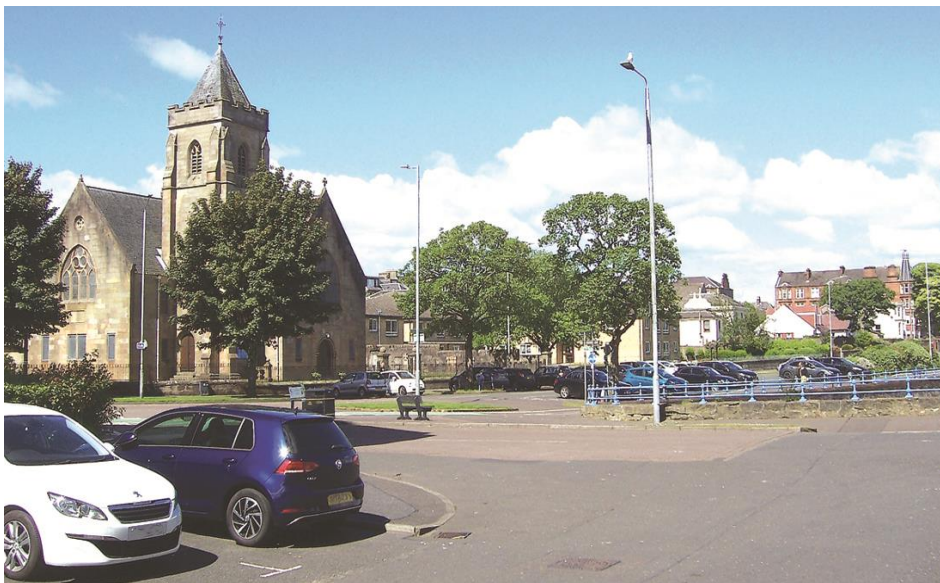
The Old West Kirk, situated at the T-junction of the Esplanade with Campbell Street, in the elegant West End of Greenock
